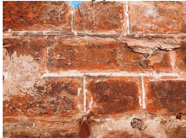
Front elevation with evidence of original wiggled brick pointing
