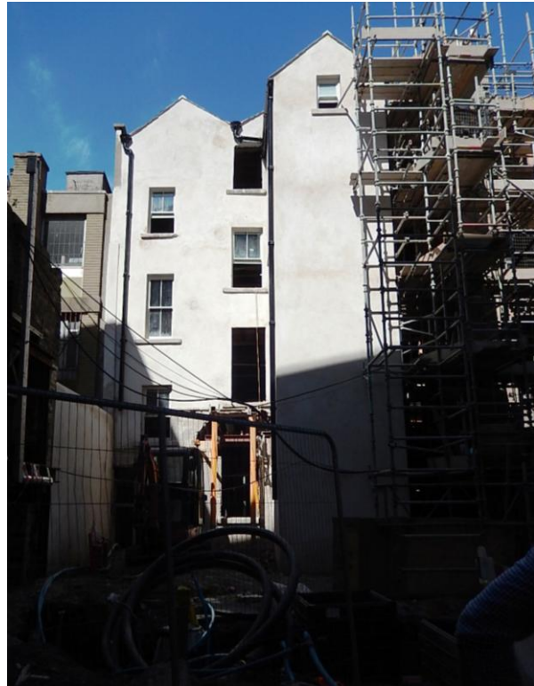
View of lime rendered rear facade
