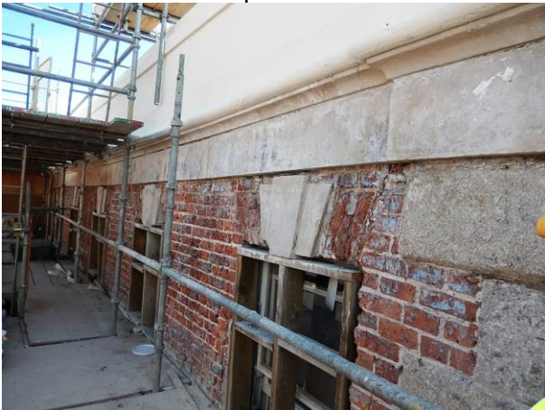
View of front elevation with original 1715 Portland cornice and keystones
