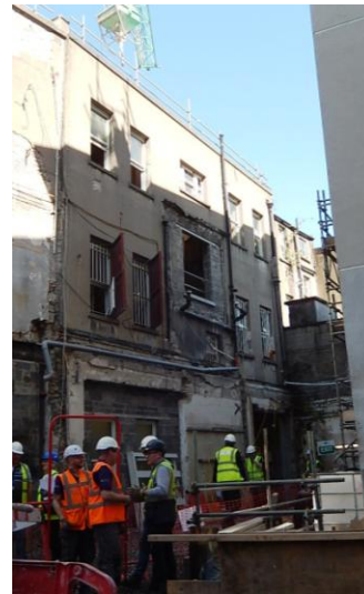
Rear elevation with largely rebuilt facade
